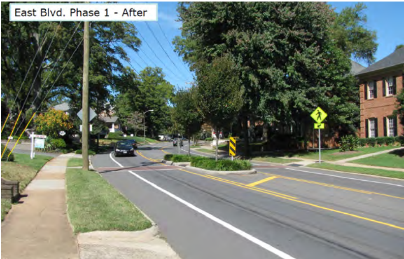
Road Diet Photo: City of Charlotte
