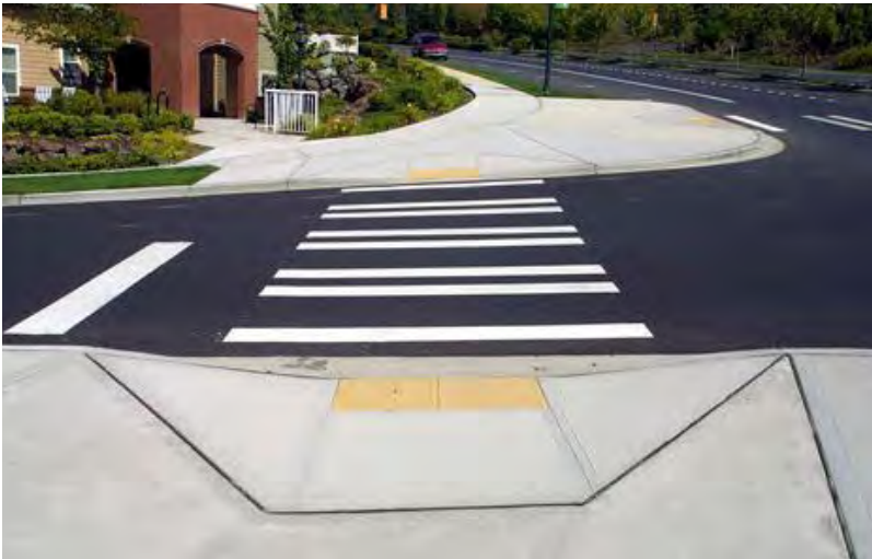
Curb Ramp Photo: NCDOT
