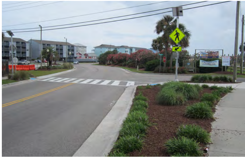
Pedestrian Signal- RRFB Photo: VHB
