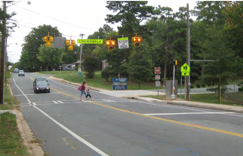
Pedestrian Hybrid Beacon (PHB) Photo: City of Charlotte
