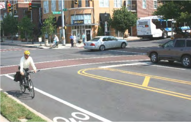
Bike Lane (Chapel Hill, NC) Photo: NCDOT
